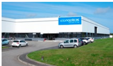
New IDEA OPTICAL factory specialising in the design and integration of optical connection and patching equipment in Lannion since August 2019. 2 out of 3 optical cabinets installed in France were designed and manufactured by Idea Optical.
