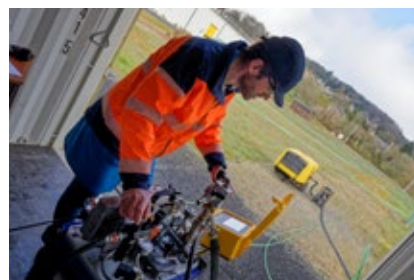
ACOME operates an optical cable blowing test centre and is developing a new blowing platform at its Normandy site.
